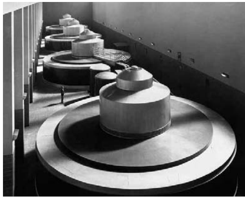
photo © National Archives and Records Administration-Southeast Region, Records of the Tennessee Valley Authority (TVA) ■ The Pickwick Dam powerhouse in Tennessee contains four generators with a capacity of 144,000 kilowatts.
